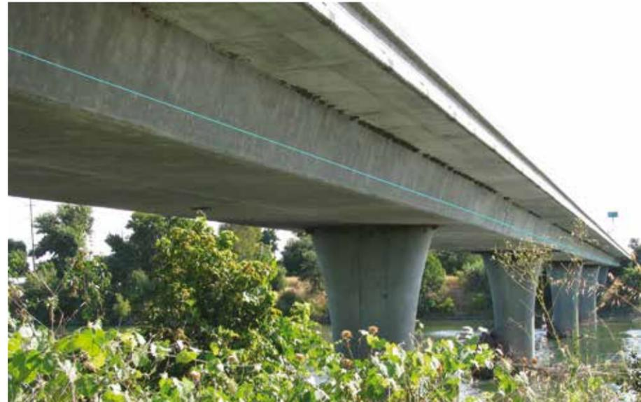
The blue line represents location of a cased span (a 10 inch diameter pipe inside a 16 inch casing) contained inside a bridge structure at a river crossing inspected with an untethered robotic MFL tool while the pipeline remained pressurised and in operation. The NT ILI tool was also run in the opposite direction away from the bridge in order to eliminate the need for additional ECDA excavations in the area.
