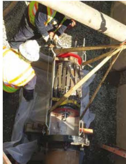
Baker Hughes' V-Line tethered MFL tool being loaded into pipeline to inspect 518 m up a mountainside in an environmentally sensitive area.
